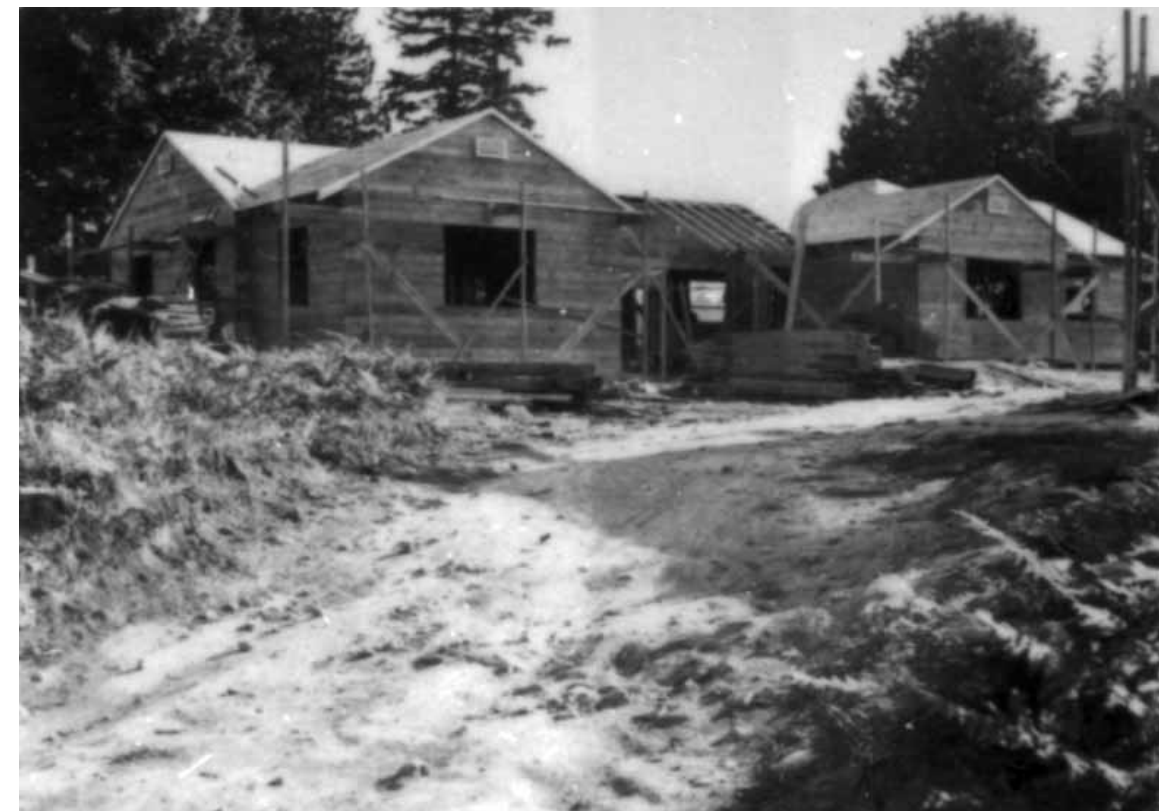
construction, 1942 [BCA BHS 370-547]
