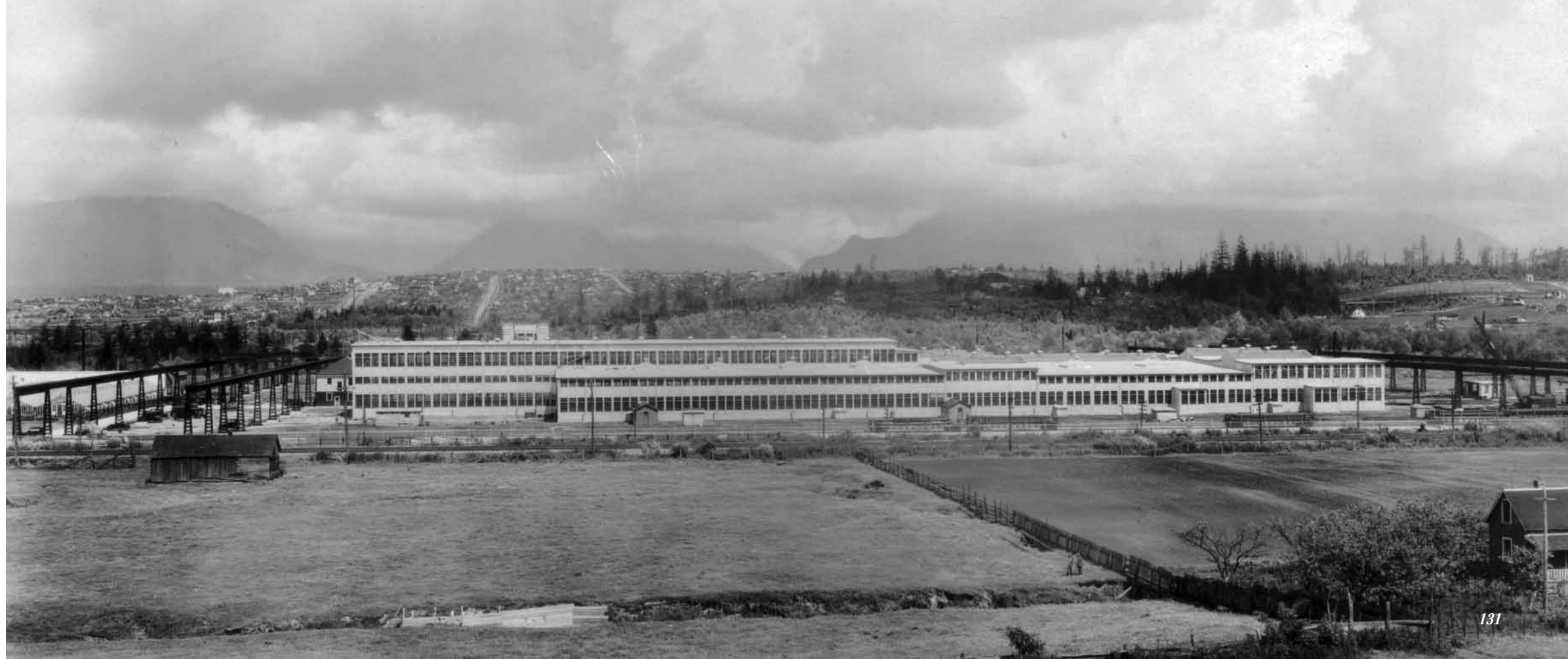
Panorama of Dominion Bridge Plant, c. 1935 [BCA]
