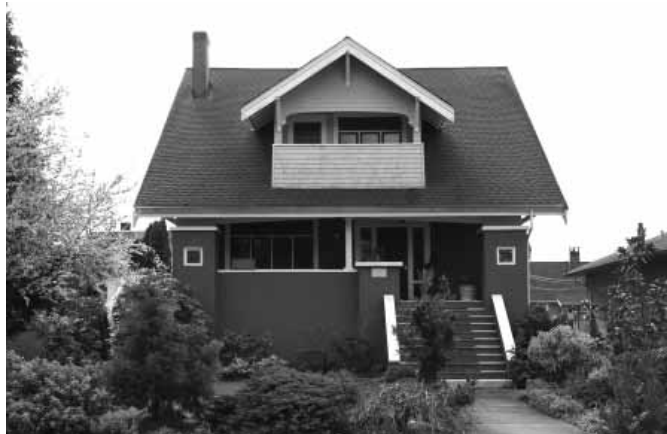
HILLCREST GEORGE & ROSE NUTTALL RESIDENCE Hillcrest 3756 McGill Street 1921
