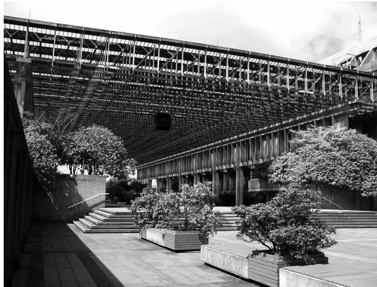
Roof [photo courtesy Steven Zhen Wang]
