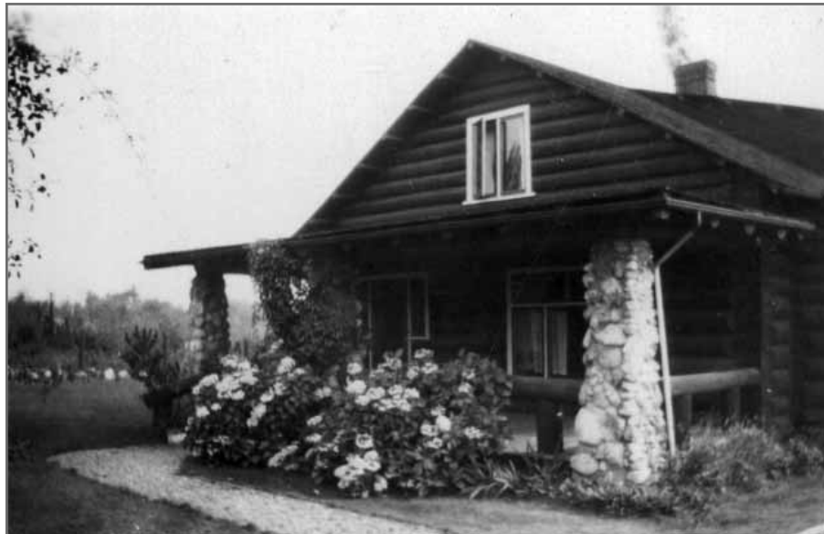
4156 Rumble Street, c. 1925 [BCA]
