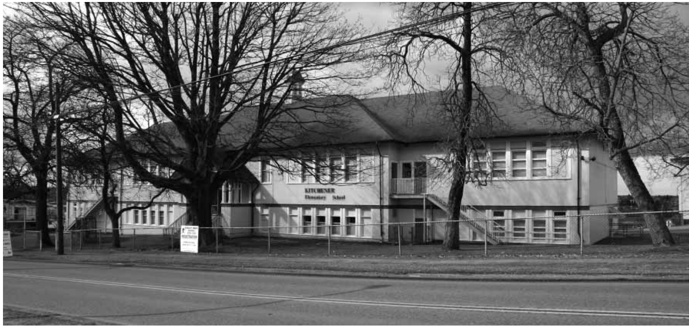
KITCHENER ELEMENTARY SCHOOL 1351 Gilmore Avenue Bowman & Cullerne, Architects 1925, 1927
