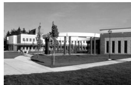
Burnaby South 2000 Secondary School
