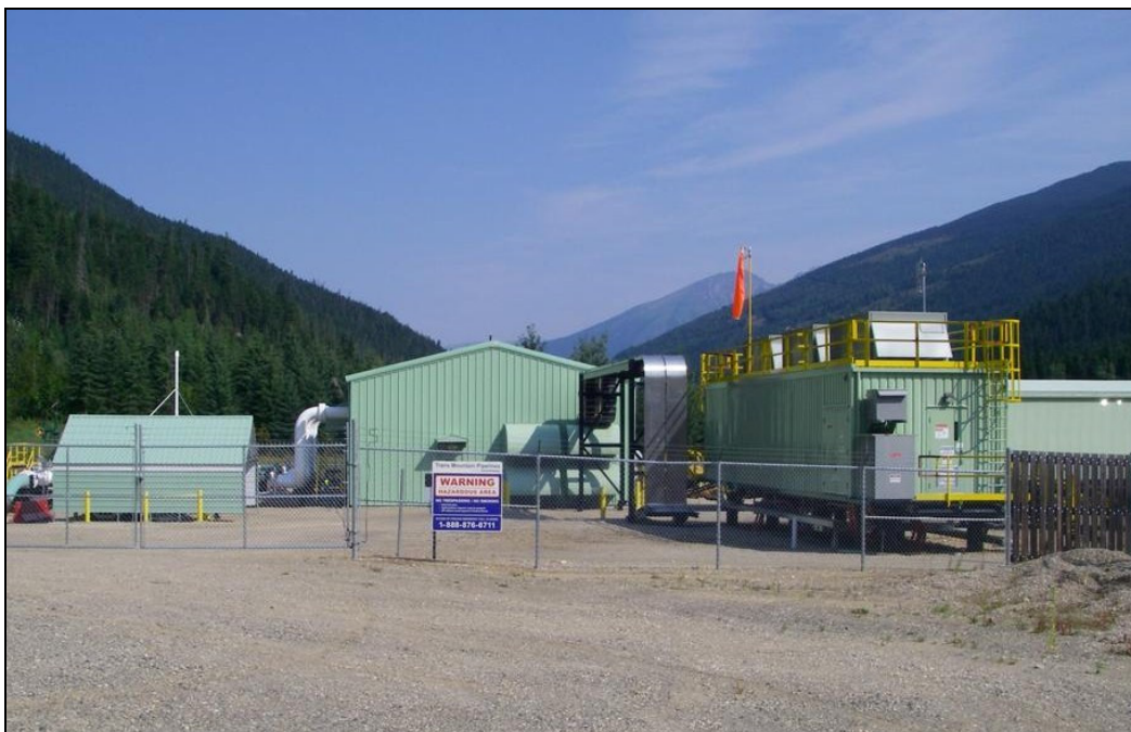
Figure 2-2: Existing Chappel, BC, Pump Station
