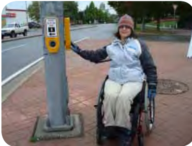
Accessible pedestrian control button.
