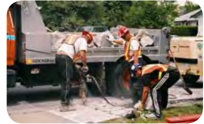
Building a sidewalk.
