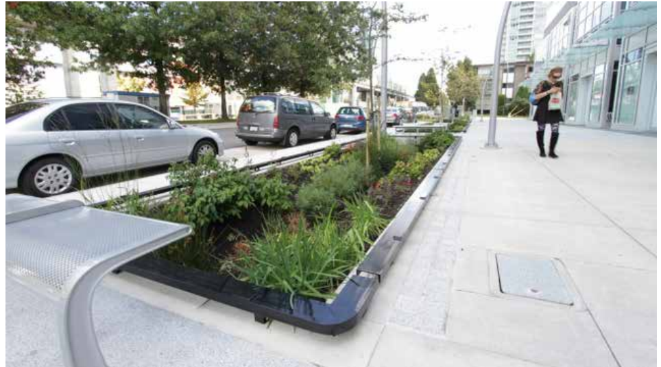
Burnaby's new street standards for town centres contribute to Burnaby being a modern-day green city by providing mobility for all, street trees/habitat, rain-gardens, and social spaces (2015 September).
