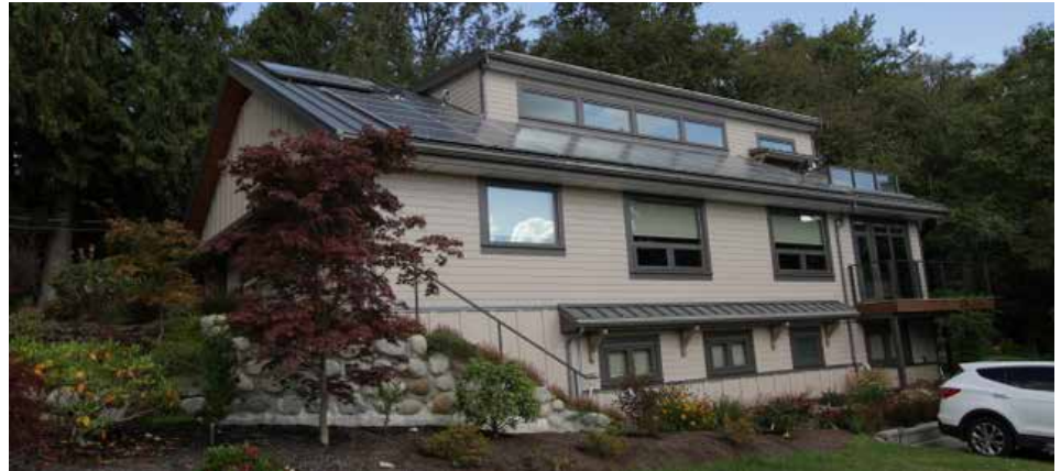
Harmony House, a single family home in south Burnaby designed to generate as much power as it uses each year.
