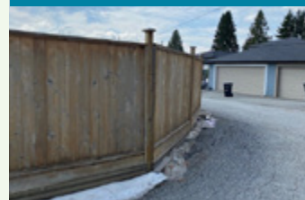
Does not meet standards: Fence blocking vision clearance
