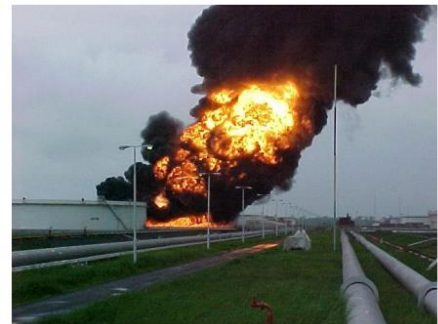
Nigeria 2002 – Note crude flowing outside bund
