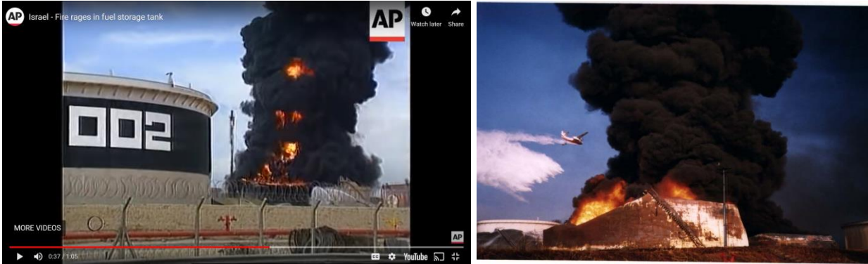
The picture above is a full surface fire example at a diesel fuel storage tank. Israel 1997
