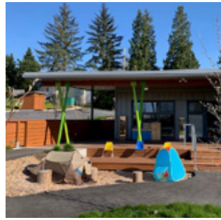
Modular facility at elementary school
