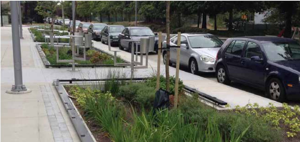
Landscaped rainwater management amenities (RMA) along the streetscape
