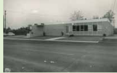
Triangle Conduit and Cable, circa 1960. This business at 7515 Gilley Avenue was one of many industrial businesses that was established in the Royal Oak neighbourhood after the Second World War. City of Burnaby Archives 112-001.
