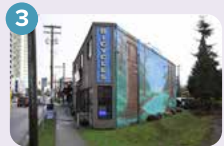
3 A triangular-shaped building where Imperial Street intersected with the interurban railway.
