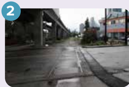
2 A track beneath Royal Oak SkyTrain Station, which serves as a reminder that the SkyTrain's route was once the Central Park Line, which connected Vancouver and New Westminster through Burnaby.
