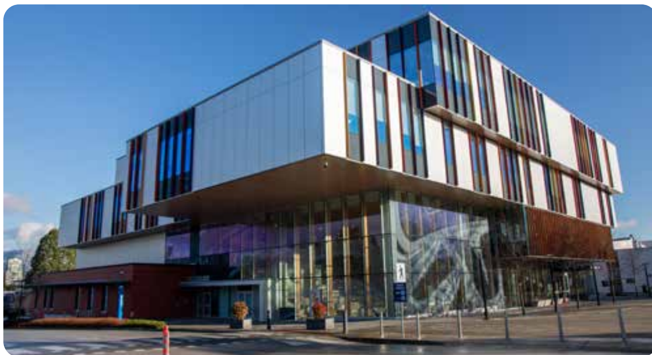
BCIT's energy efficient Health Sciences Centre
