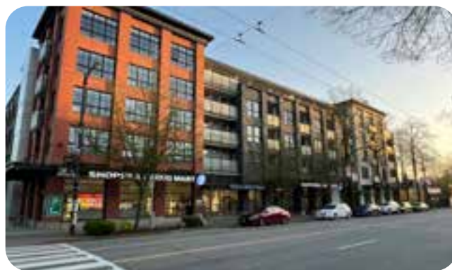
Mixed-use buildings with commercial units at ground level and apartments above
