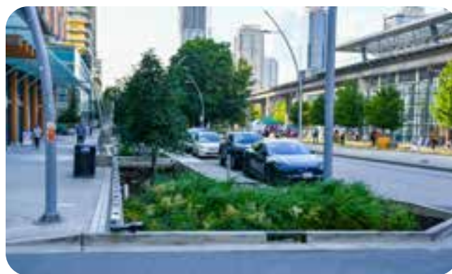
Raingardens along Beresford Street
